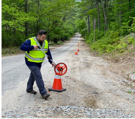
HSEM's Austin Brown assists with a preliminary damage assessment after flooding in spring 2023.
