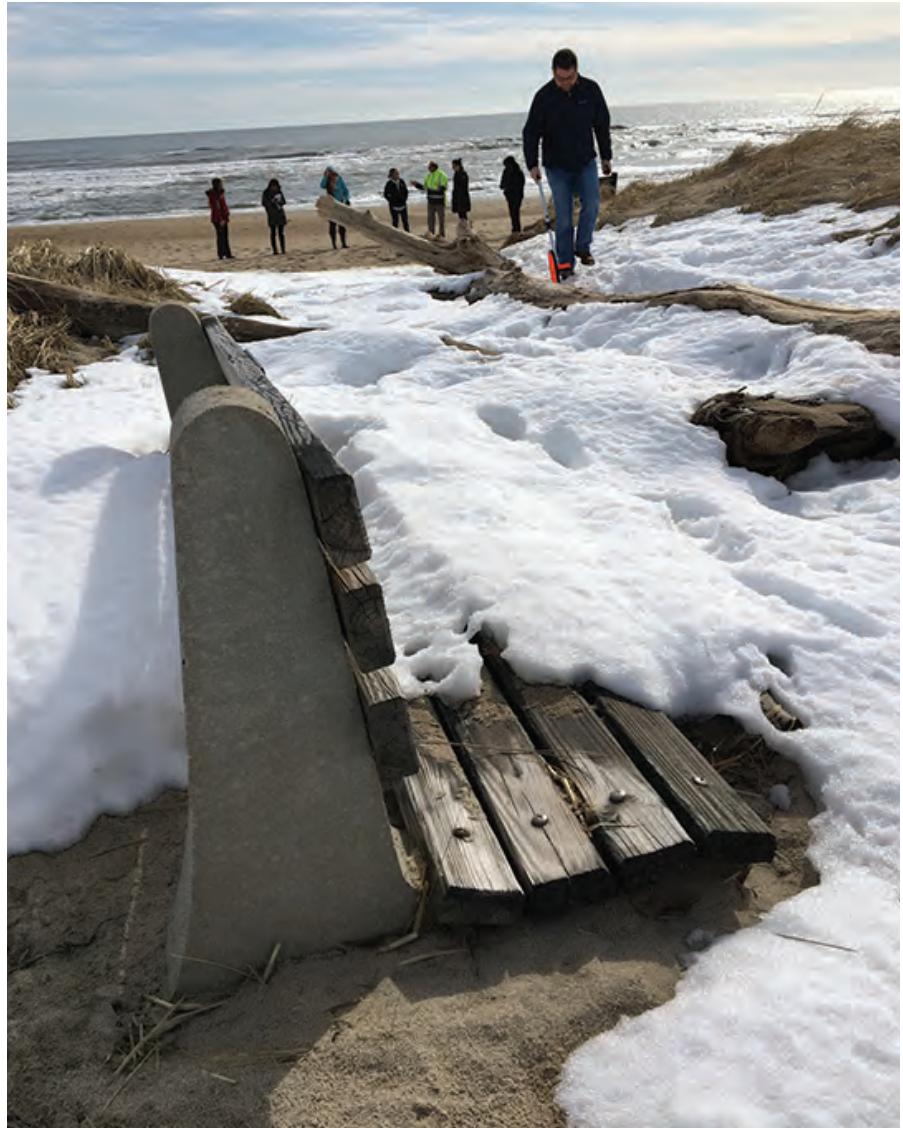
ABOVE: HSEM and FEMA staff conduct a preliminary damage assessment in Rye following a storm in March, 2018. Field Services provides technical and organizational assistance in preparing for, responding to, mitigating and recovering from natural, human-caused, technological disasters and emergencies.
